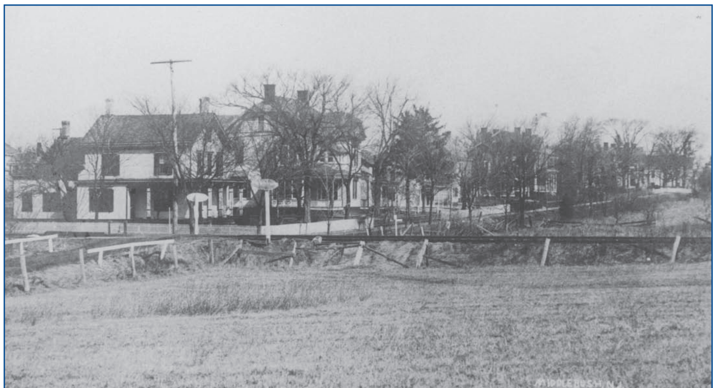
Railroad Crossing at South Middlebush Road, looking north, (c.1908)
