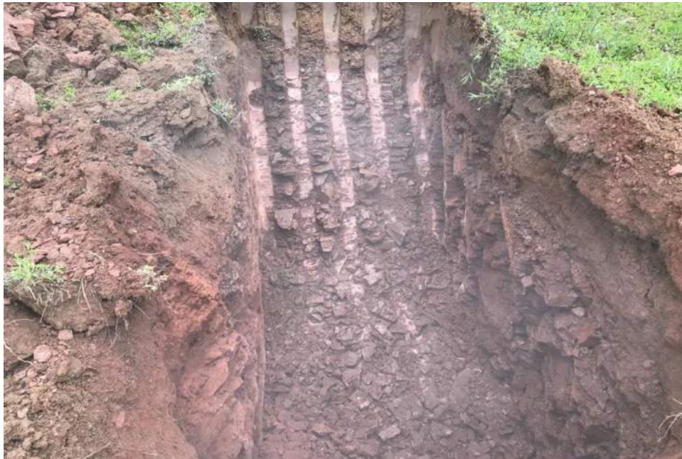
Photo 38: TP-217 Profile pit
