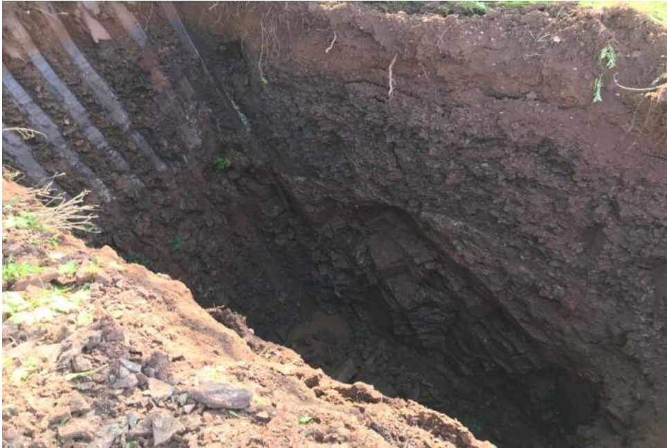
Photo 7: TP-104 Profile pit
