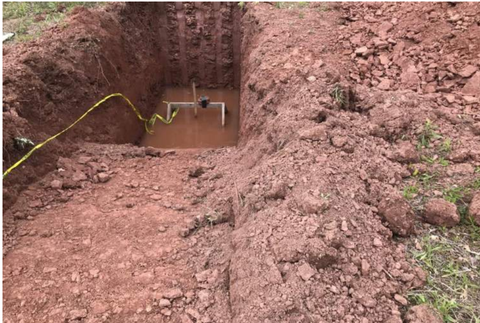
Photo 22: TP-202 Basin Flood Test set up
