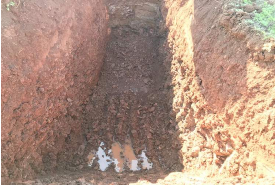
Photo 8: TP-105 Profile pit
