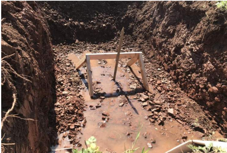
Photo 6: TP-103 Basin Flood Test set up
