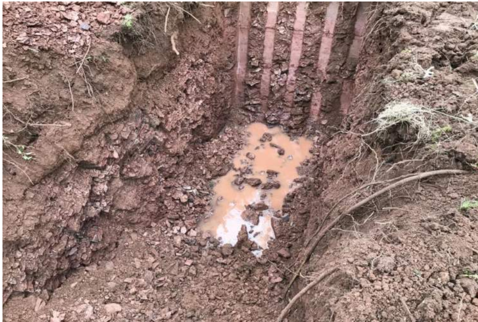
Photo 18: TP-114 Profile pit
