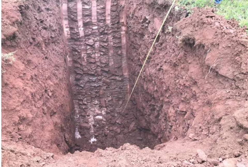
Photo 37: TP-216 Profile pit
