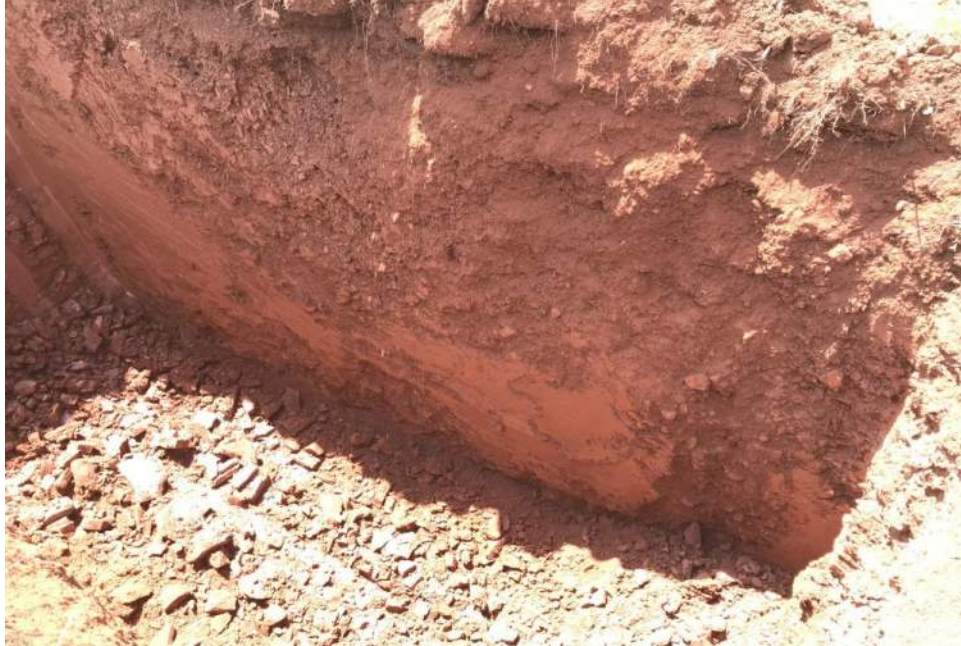
Photo 31: TP-210 Profile pit
