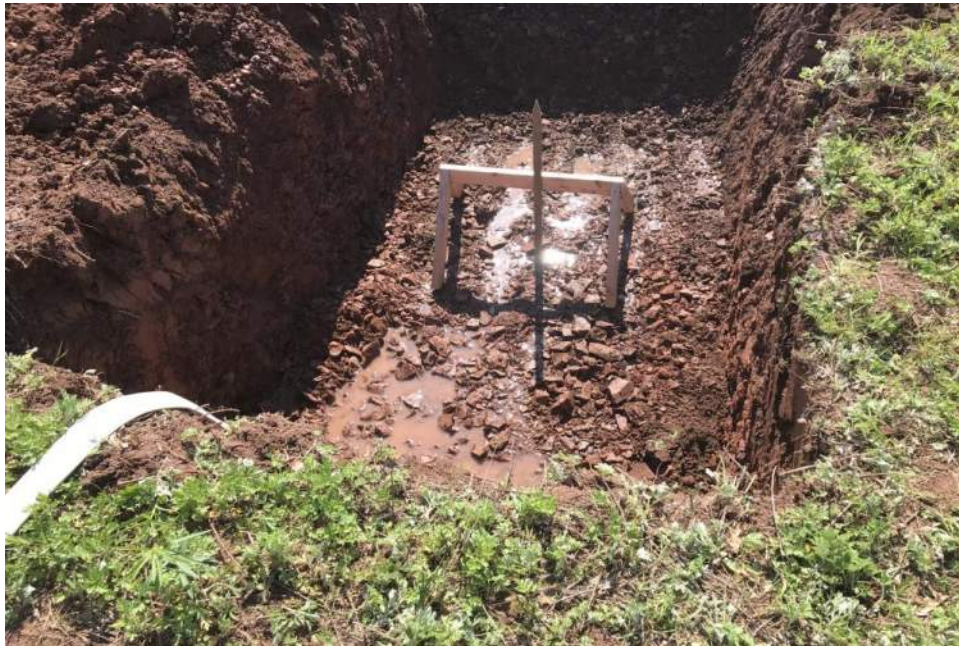
Photo 2: TP-101 Basin Flood Test excavation and water seepage
