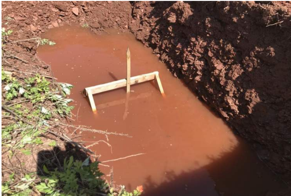
Photo 4: TP-102 Basin Flood Test set up
