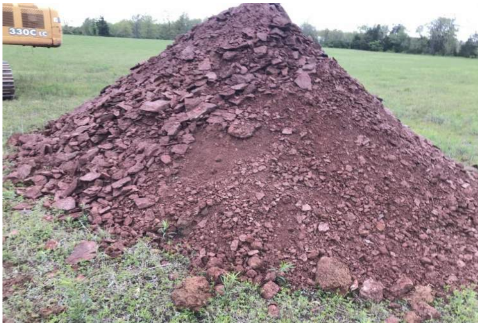
Photo 40: TP-218 Excavated material
