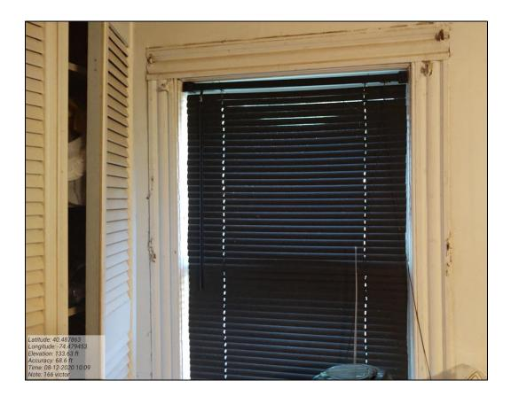
This one of several interior windows, each with casing (the trim around the window) of the size and style commonly used from the 19<sup>th</sup> century though the 1950's.
