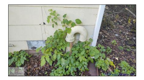
This is a 4" cast iron sewer vent on the exterior of the building. Cast Iron was used though the 1960's and started to be replaced in new construction in the 1970's by various plastic pipes. Cast iron was commonly used in the 1950's as it replaced the often-used clay and transit pipes of the early 20 th century.
