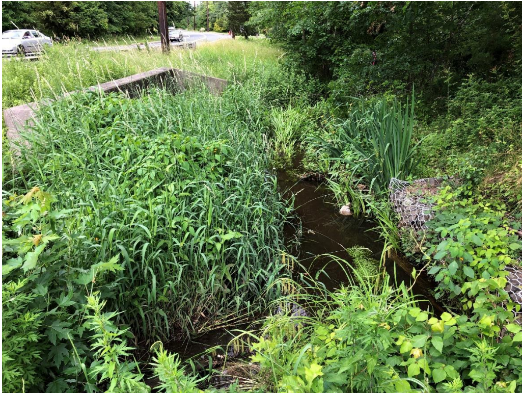
Existing headwall at Elizabeth Avenue where tributary enters the Site.
