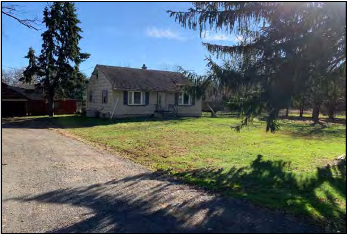
Photograph facing south from the northwest corner of the property boundary, showing the single-family residence located at 471 Elizabeth Avenue.
