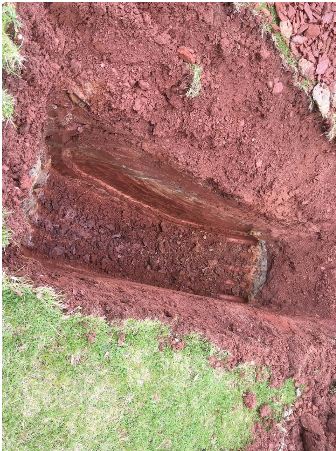
Photograph 7 – Test Pit TP-109
