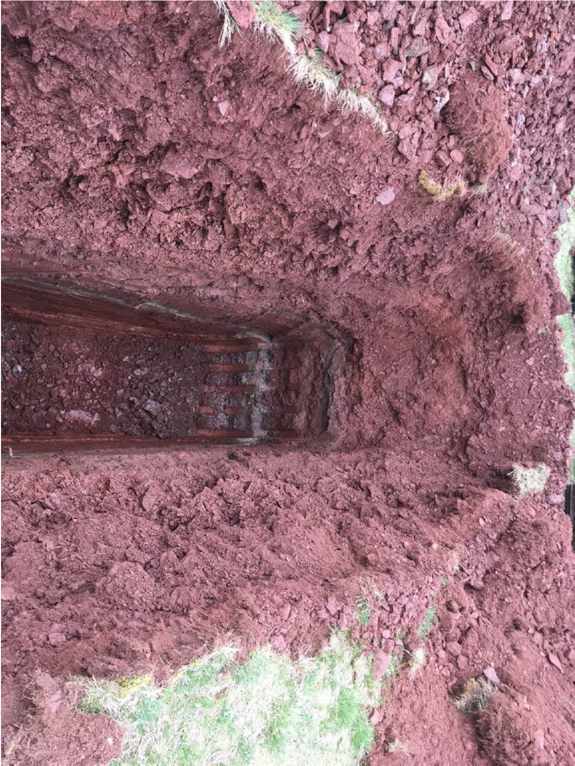
Photograph 2 – Test Pit TP-102
