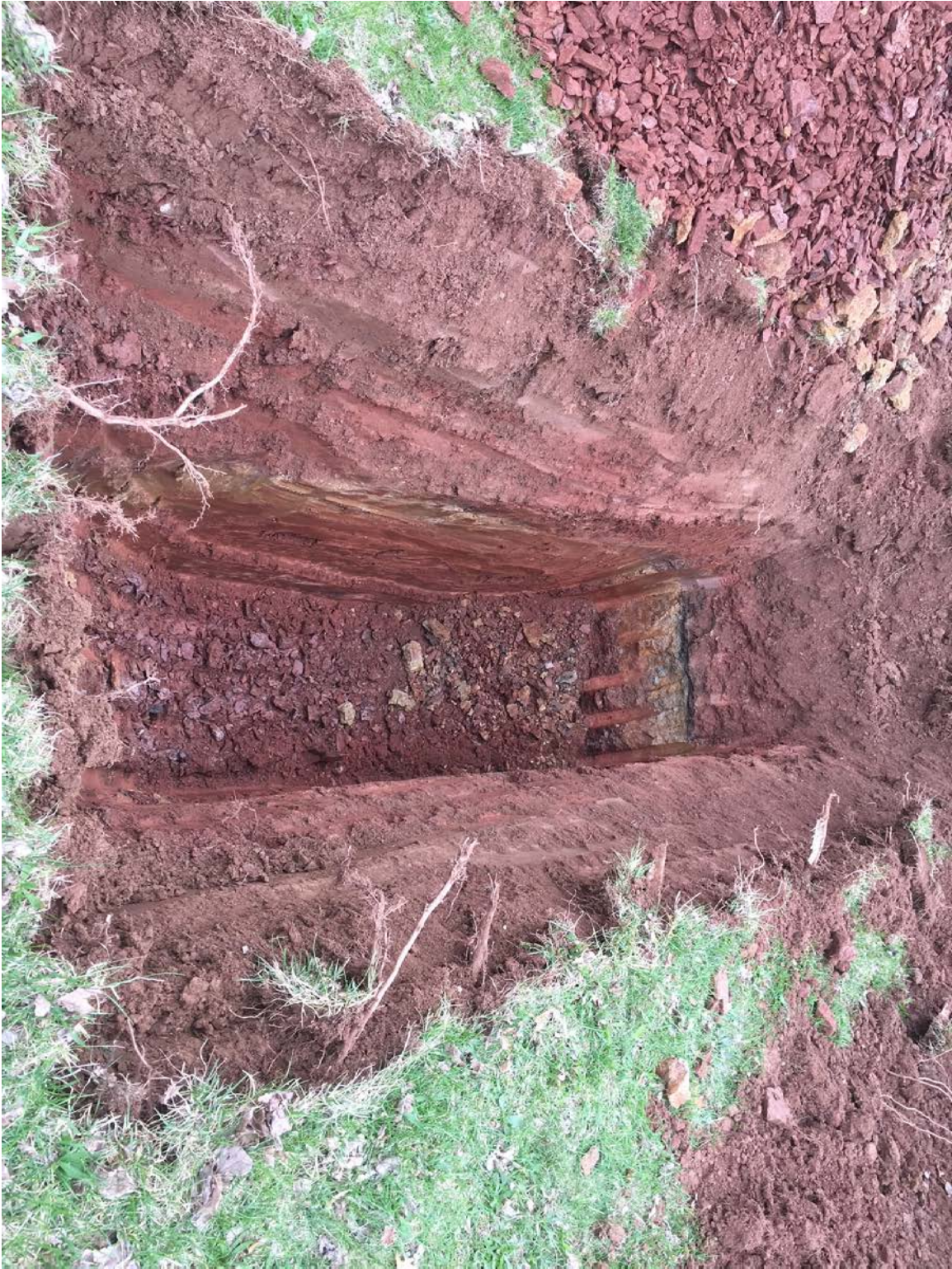
Photograph 3 – Test Pit TP-103
