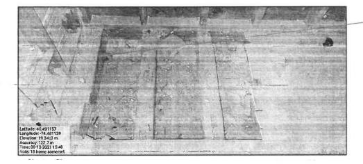
Floor joists of fullsized lumber, indicating pre-1940s manufacture
