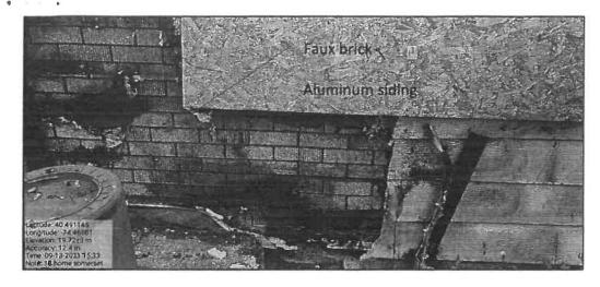
The fibrous imitation brick siding may be the original siding because it was popular in the area from the 1920s through the early 1950s. Along with the other components of this building, this supports a 1950s or early construction and occupancy. The aluminum siding was likely installed in the 1960s or early 1970s.
