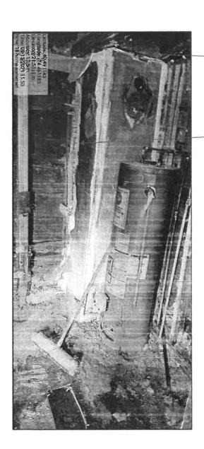
The chimney is framed as part of the original construction. The use of a full sized chimney indicates the intention of occupancy.
