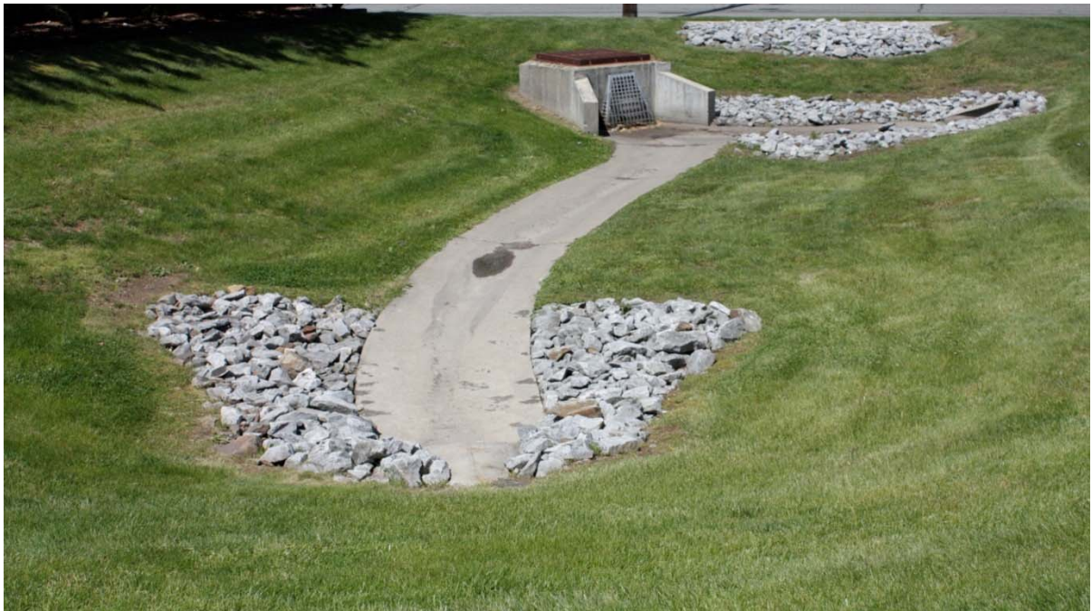
A well maintained detention basin
