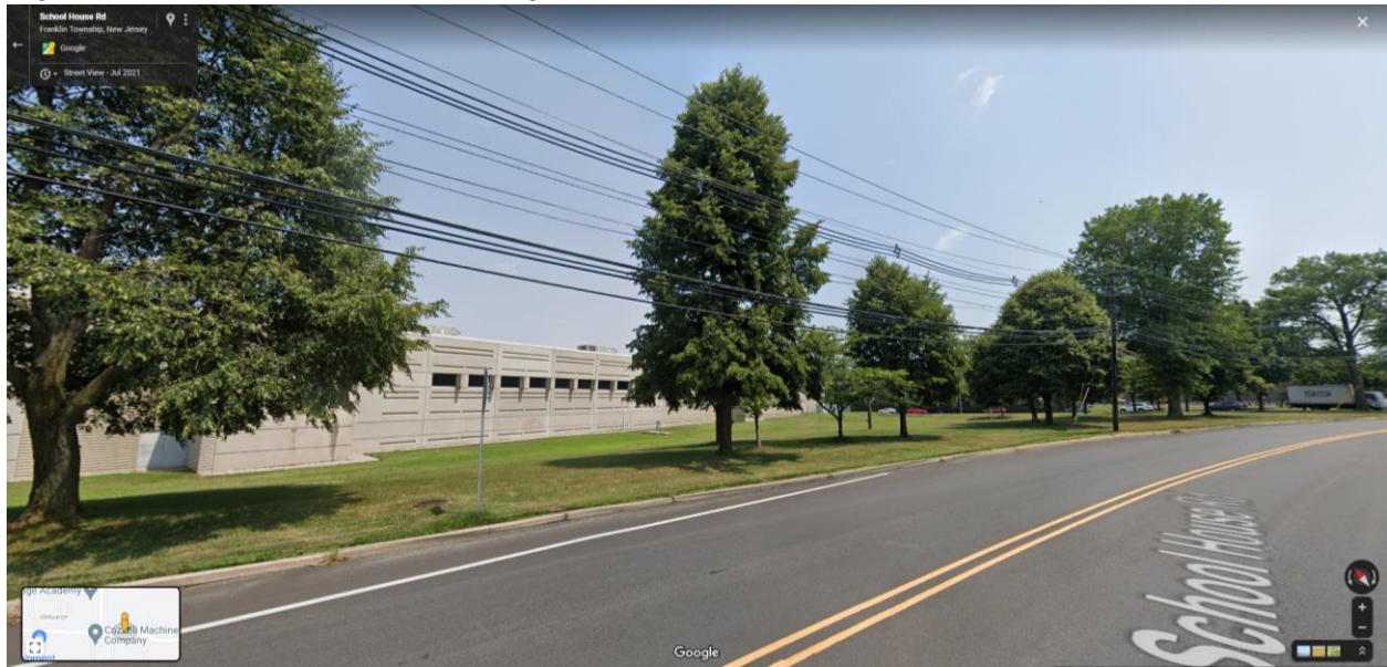
Figure 3: School House Road frontage
