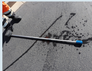
Wand used to loosen debris
