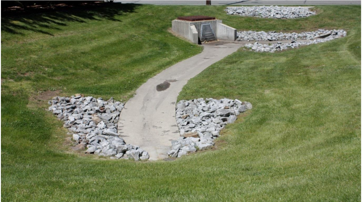
A well maintained detention basin
