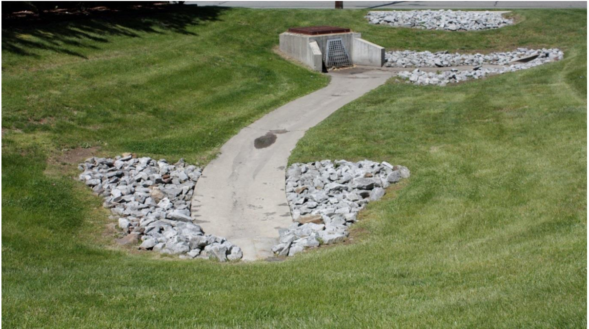
A well maintained detention basin
