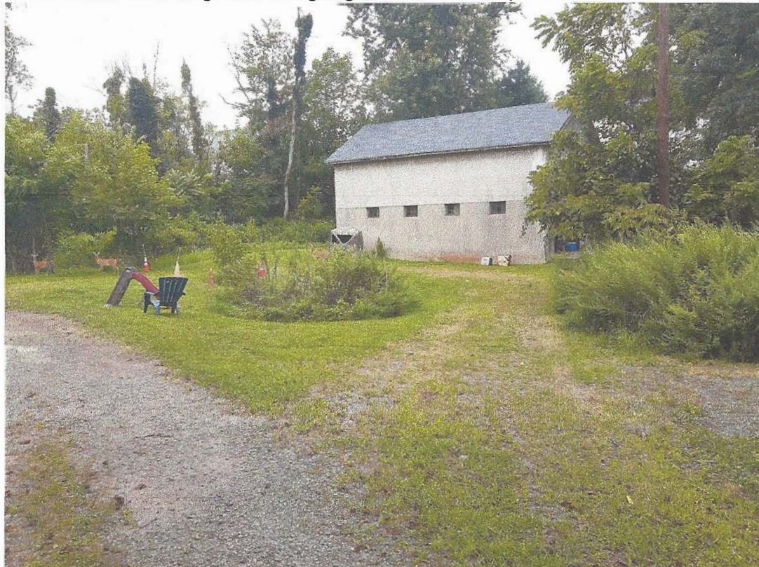
Photo 4: View of existing barn in northwestern portion of the site.
