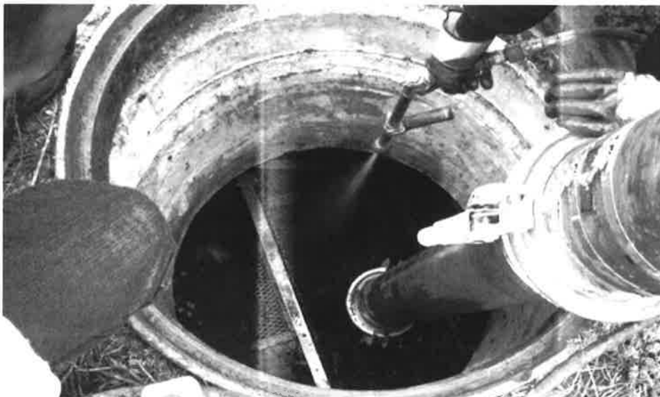
2. Insert vacuum hose in the sedimentation chamber and vacuum out all trash, sediment and standing water.
