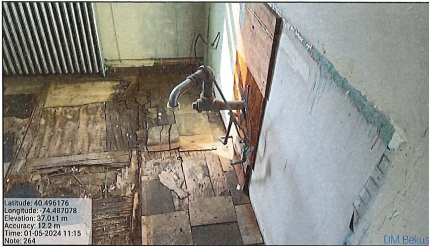
Basement kitchen cabinets have been removed.
